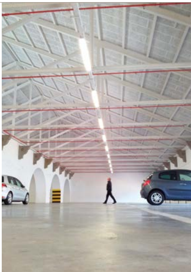
SILOS PARKING Trieste, IT photo: Eddy Tiozzo
