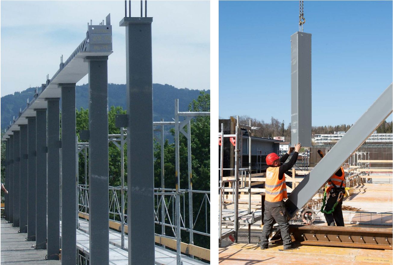
Figure 7. Installing ATLANT® Family columns on site.
