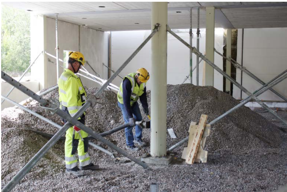
Figure 12. Concreting from bottom, revision of proper filling must be done at top end.
