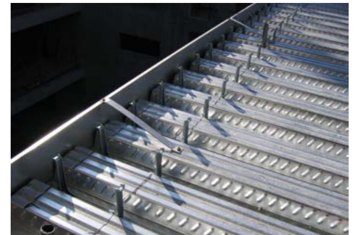
Edge trim with restraint strap and nailed shear studs
