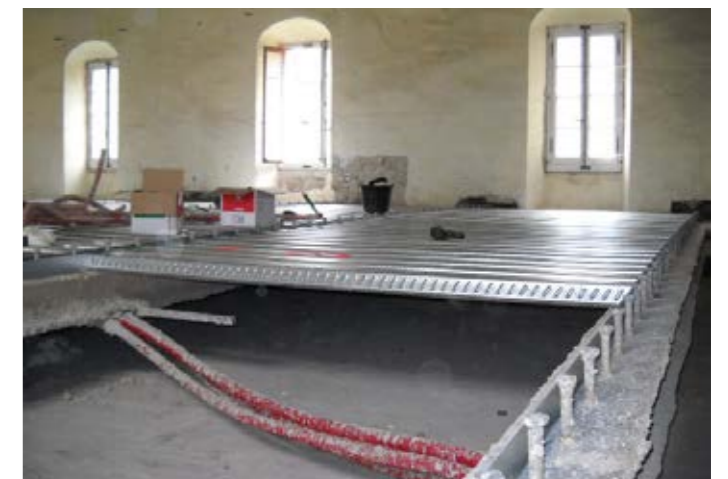
Installation within rehabilitation project - Cofraplus® 60
