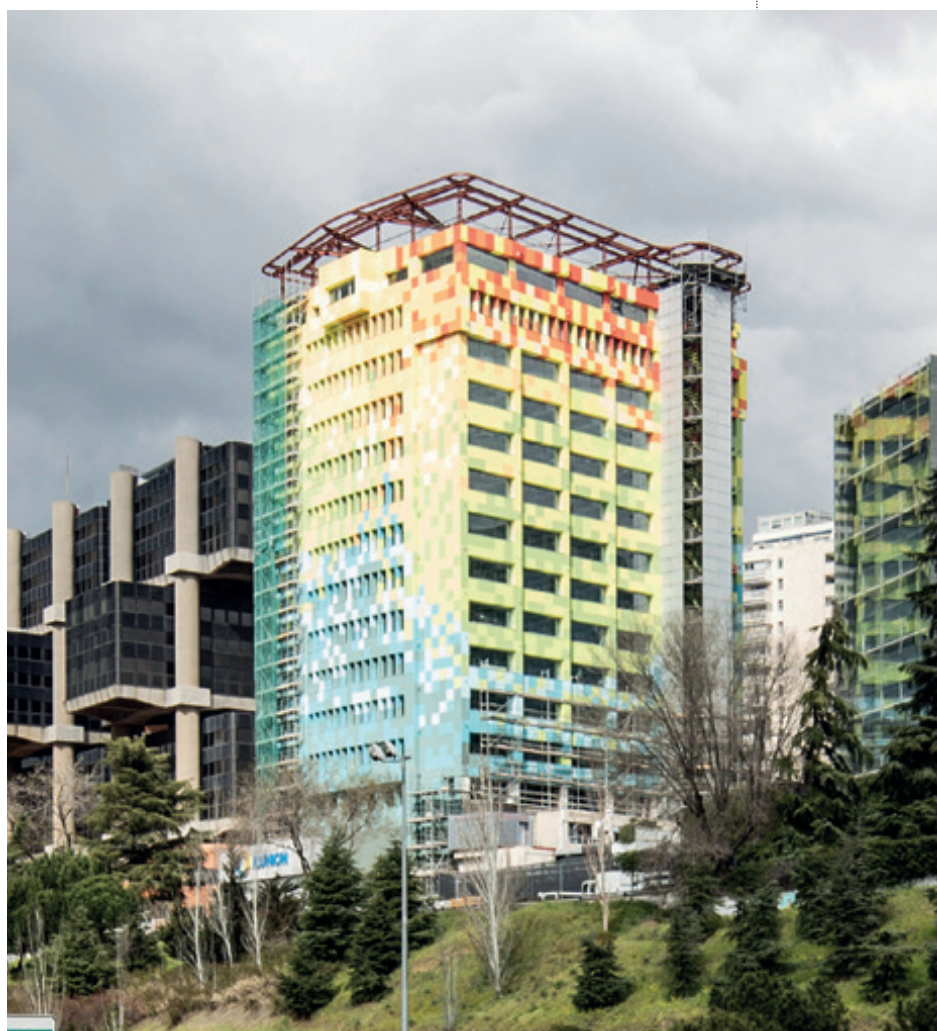
#4 PROJECT Torre 30 – First skin Madrid, Spain
