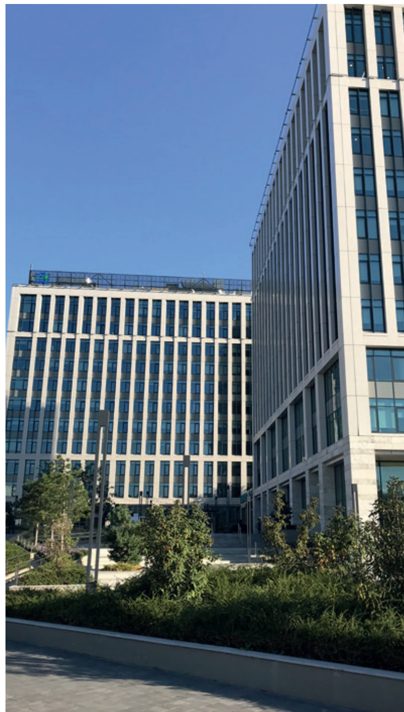
#2 PROJECT Timpuri noi square 1 Bucharest, Romania
