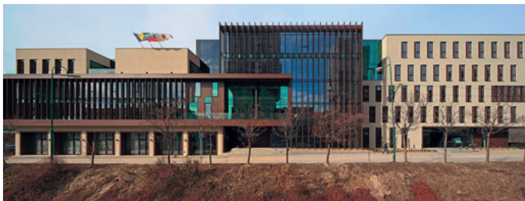
#1 PROJECT Municipality Kakanj Kakanj, Bosnia & Herzegovina
