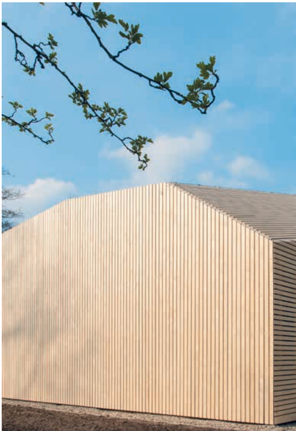
BOILER HOUSE, AMSTELVEEN, THE NETHERLANDS
